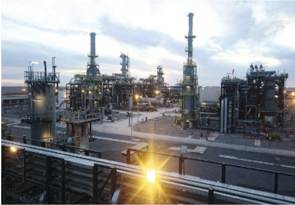
FIGURE 1.3 – Vue de la zone process du CPF (Central Processing Facility)
