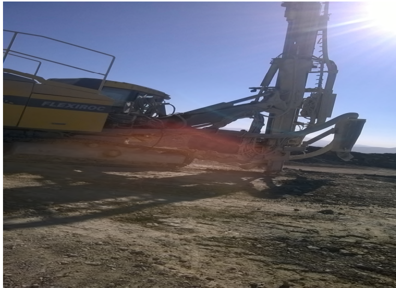
Figure III.5 Foration d'un trou de mine.
