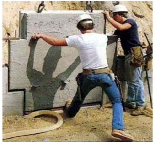
Figure I.4 : pose de la "peau"
