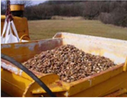
Figure 6-2 Ballast (gravier roulé 15/30 mm)
