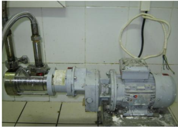
Figure I.9: Pompe centrifuge
